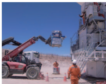
Installation of the receiver in the antenna
