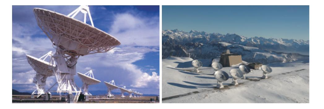
Left: The Karl G. Jansky Very Large Array (VLA) at Socorro, New Mexico, is an array of 27 antennas with diameters of 25 meters. Since its dedication in 1980,
