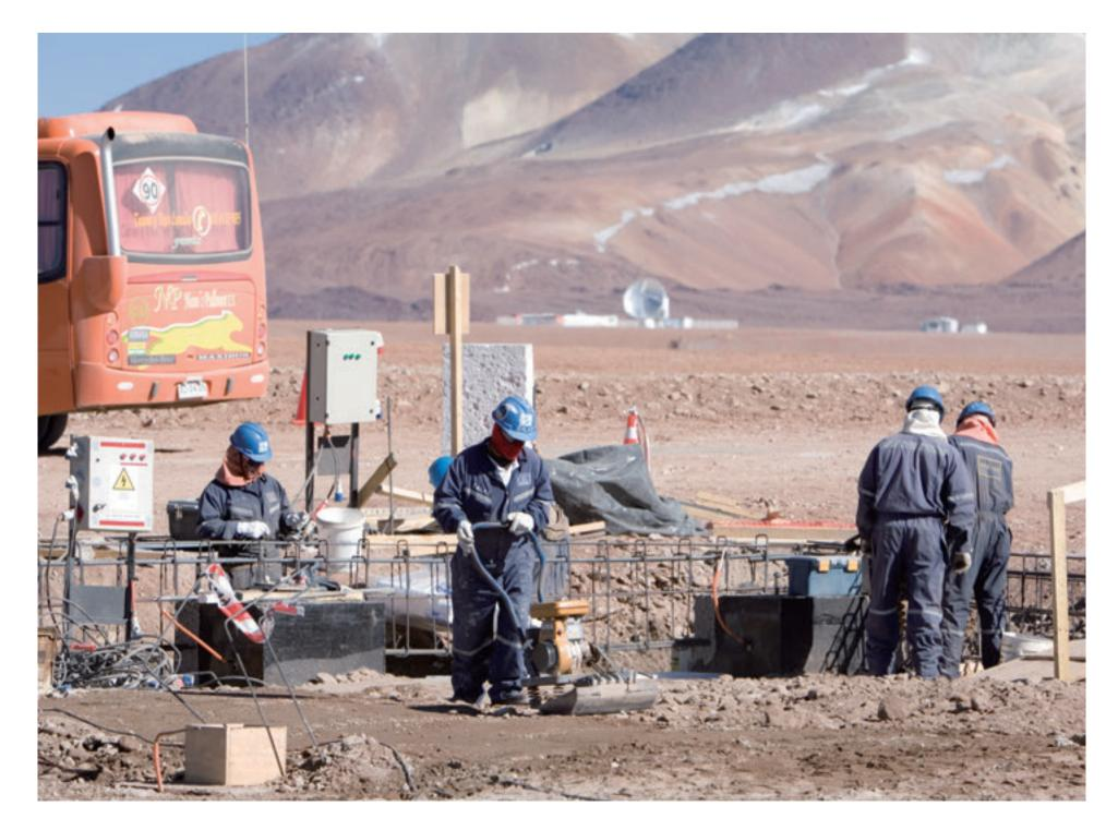
Construction of an antenna foundation at AOS. The antenna behind the workers is the Atacama Pathfinder Experiment telescope, APEX, operated by ESO. Credit: ALMA (ESO/NAOJ/NRAO)
